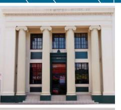
Metcalfe Constructions were engaged to rectify the foundations and repair all visual damage to the external façade of the old Commonwealth Bank building in Maryborough and restore the building to its' original condition.
